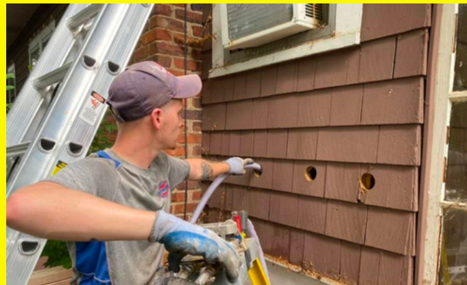
Figure 2. Insulation injections are non-invasive
