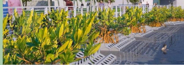
Fig 1: SEAHIVE With Concrete, Mangroves and Corals for Natural Protection
